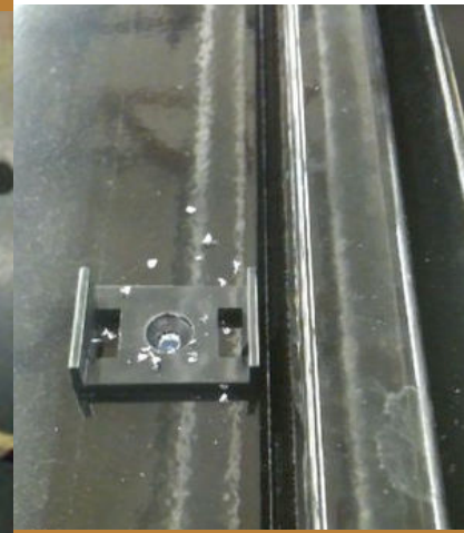
Screw in Flat Metal Clip or Roto Clip onto "Eye Brow"
