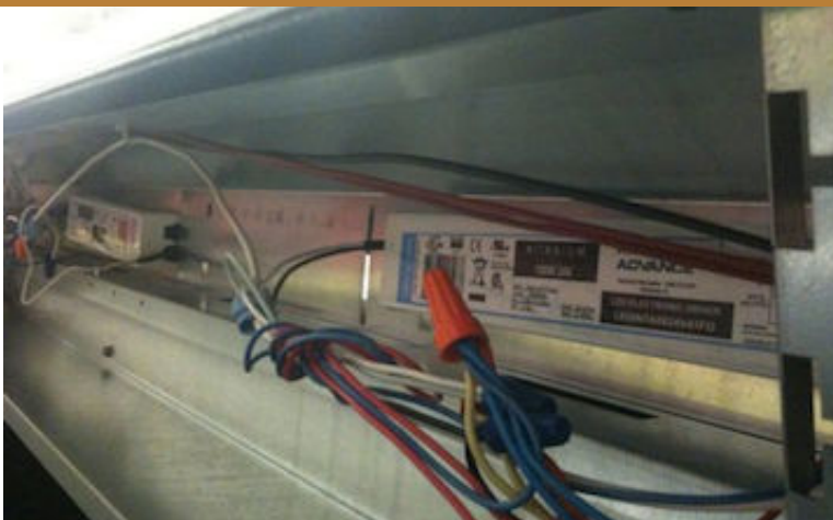
Mounting Power Supply in the Electric Raceway
